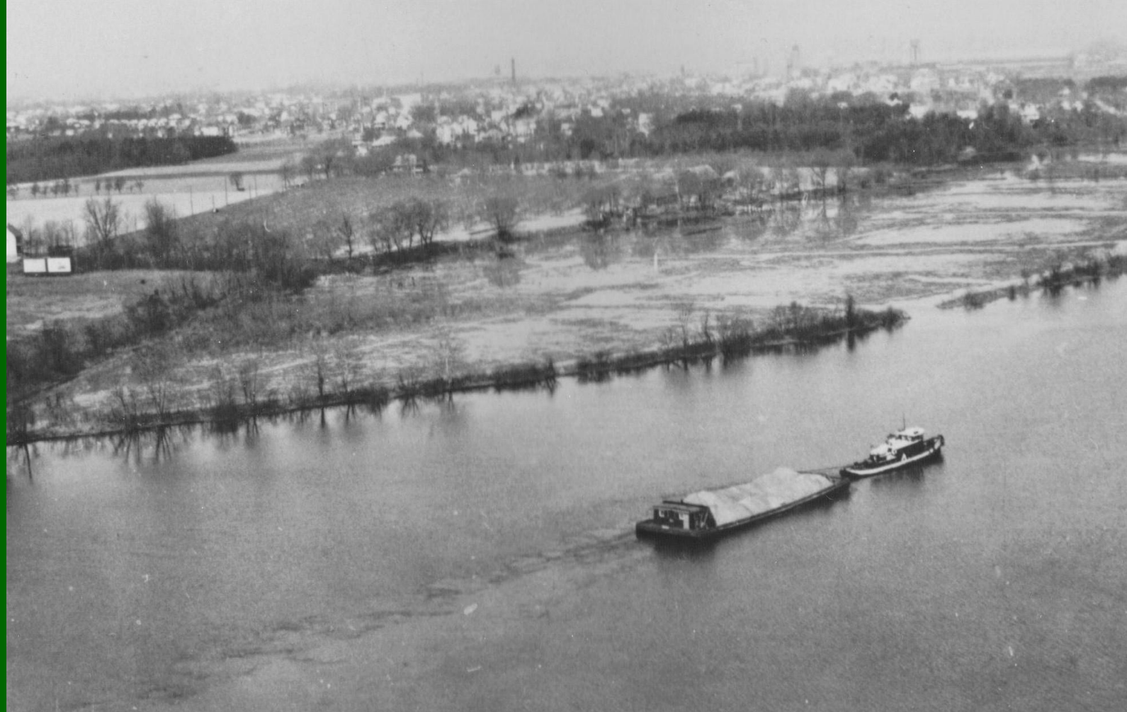
Rancocas Creek Tethered Barge Reference: Tracy Muller Photo
