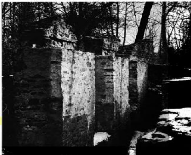
Foundations of mill building along an old raceway
