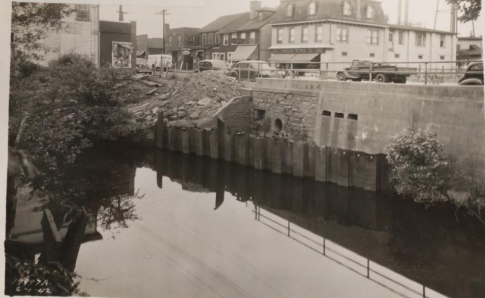
Flood Protection Works at Mt. Holly, N. J. Contract No. W-697-eng-3460. Contractor: Foundations & Excavations, Inc. 1937 - Temporary cofferdam at south end of by-pass channel - camera on Mt. Holly Textile Co. bridge, facing northwest.
