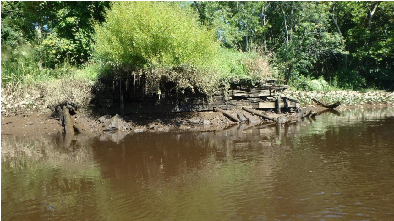
Figure 16 Existing bulkheading and dock structure designated for maritime use of some type.
