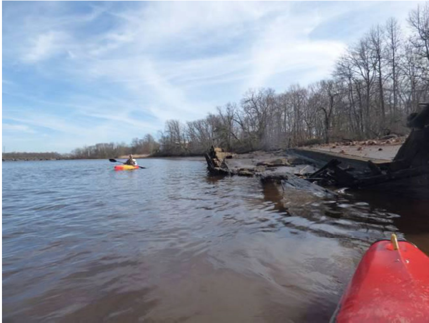
Figure 25 Remains of barge and loading dock alongside the creek for phosphorus works.
