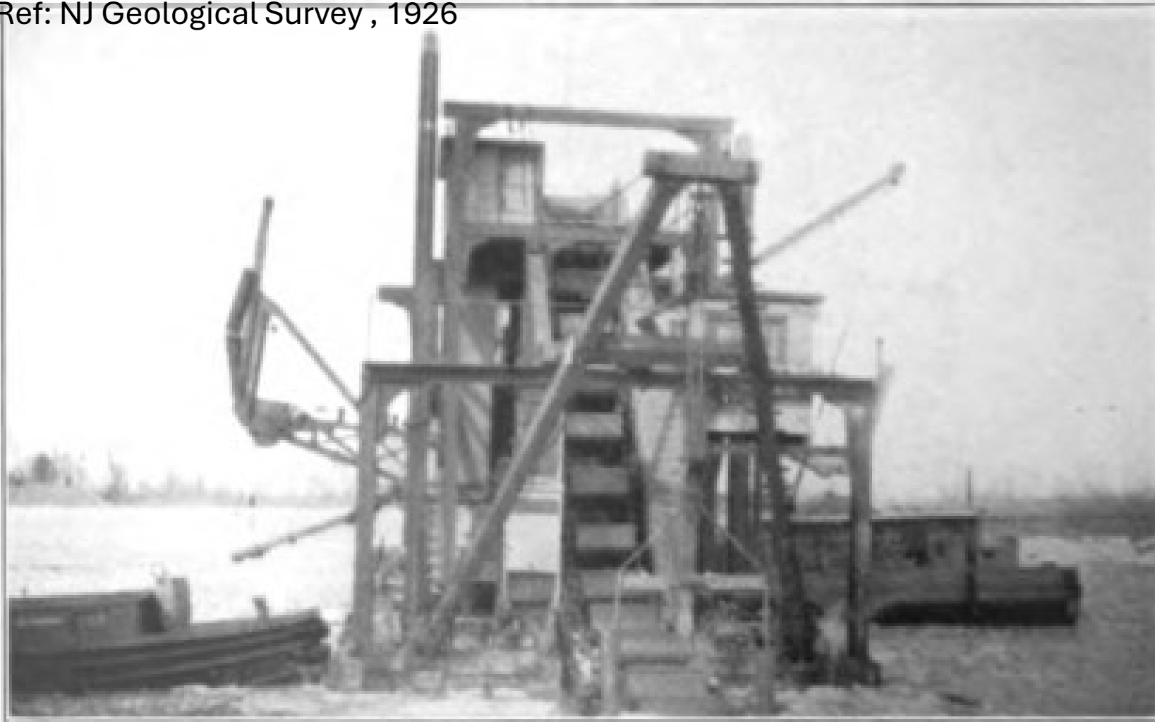
(b) River dredge operated by the Warner Company in Delaware River below Riverside, Burlington County.
