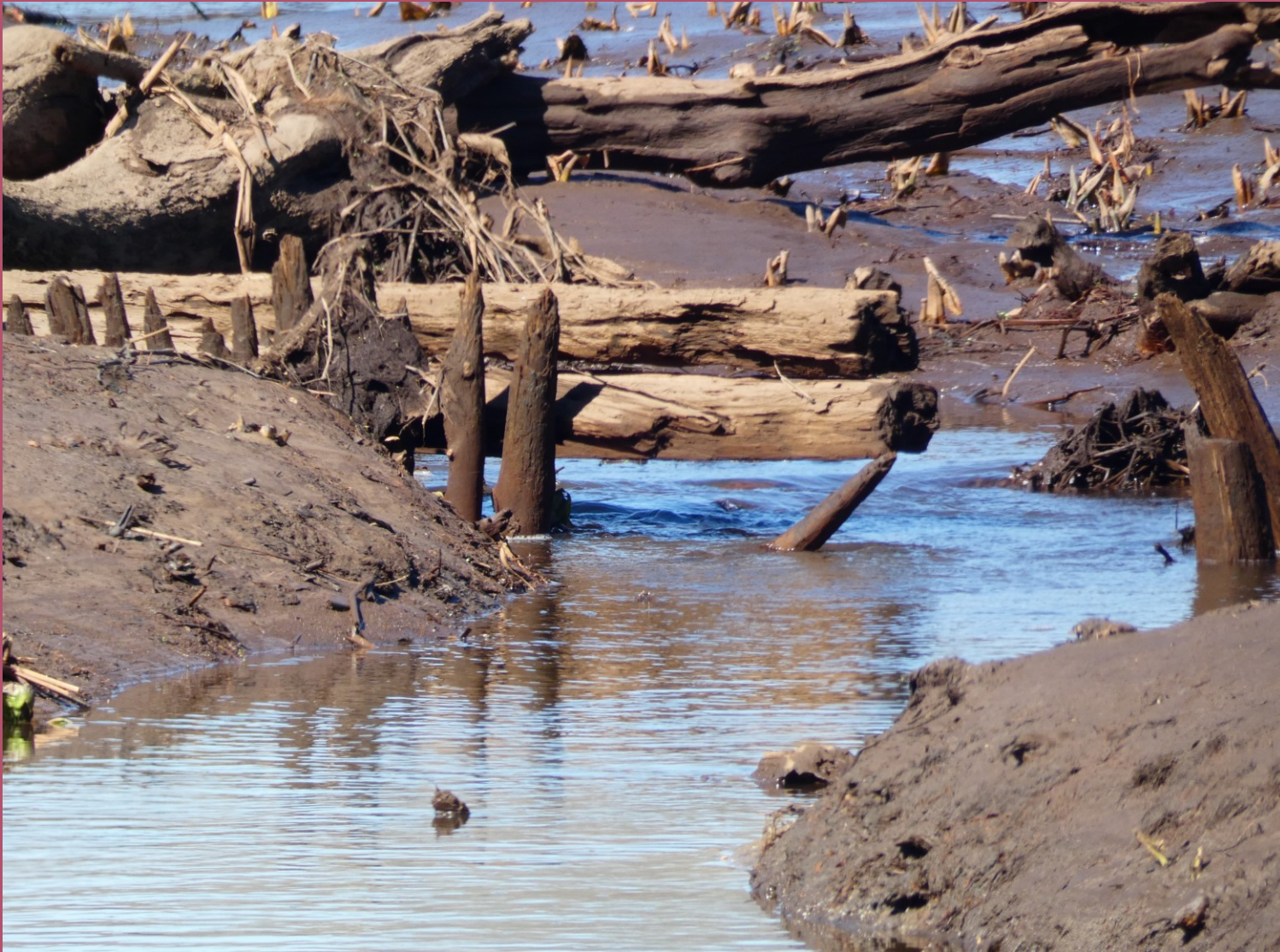
Tide Gates Cast Away Island
