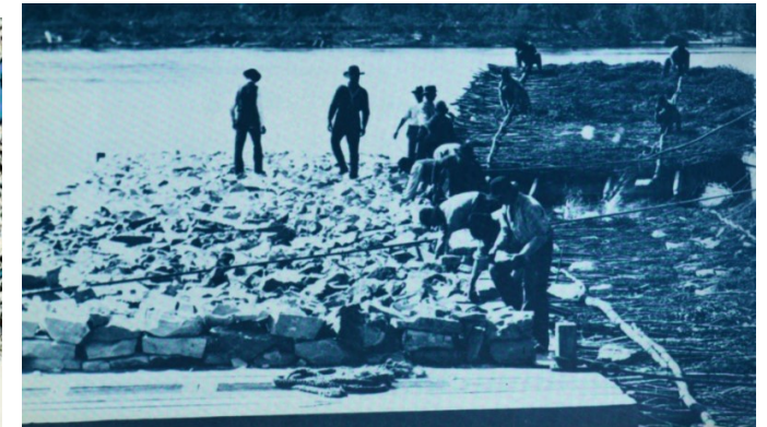
An example of an early 1900's navigation chart showing wing dams and constructing a wing dam on the Upper Mississippi River Channel. Wing dams are constructed of stones and brush.
