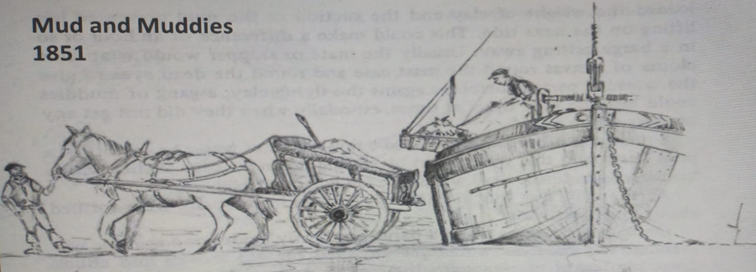
Extraction Method for Clay/Sand Holes Along a Tidewater Creek/River (as an example)
