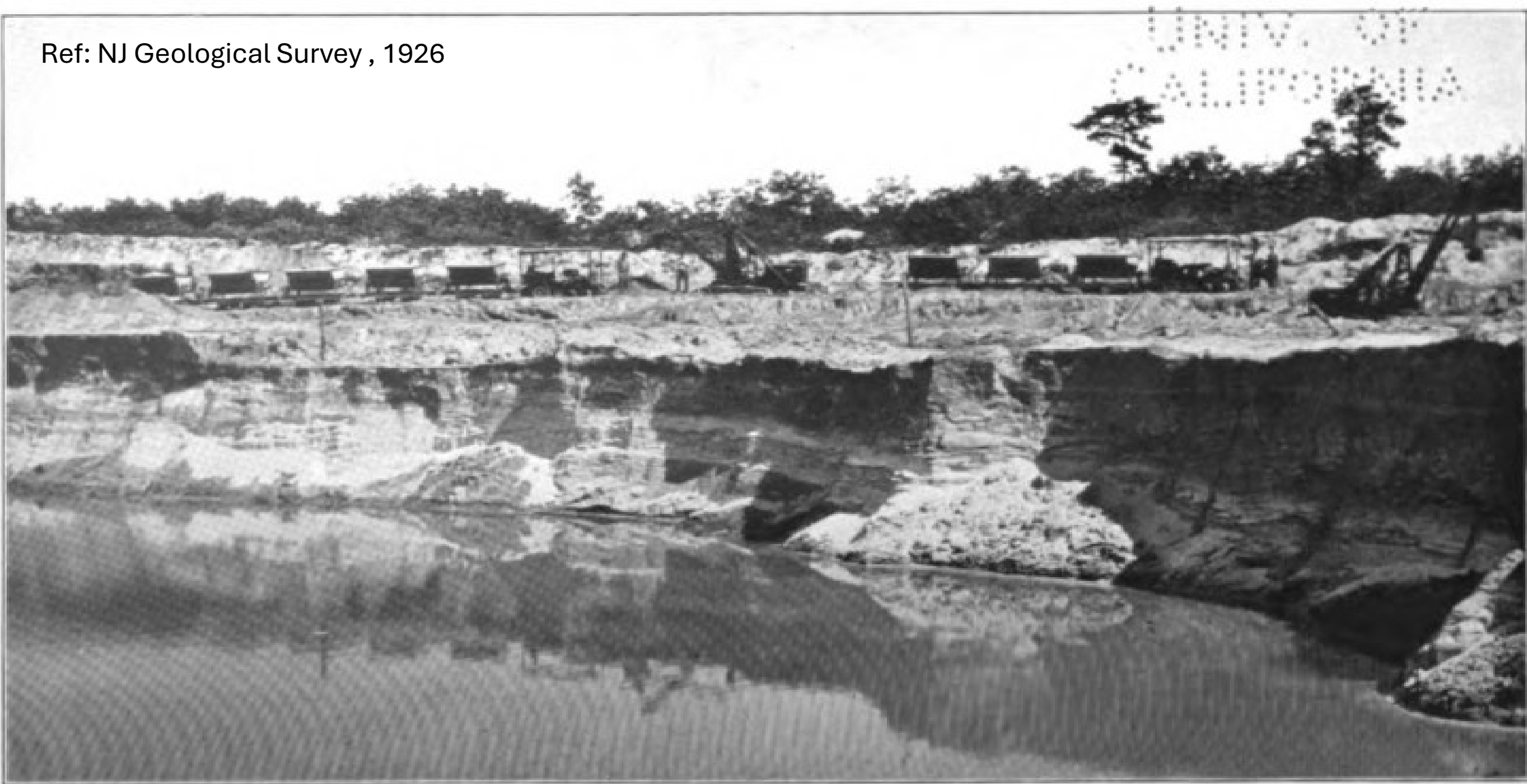
Sand pit near Manumuskin, Cumberland County. Well-bonded molding sand is dug from above the steep bank and carried in the cars shown to a railroad loading station. "Sharp" sand for foundry use is dug from the lower bank by a dredge operating in the pond shown.
