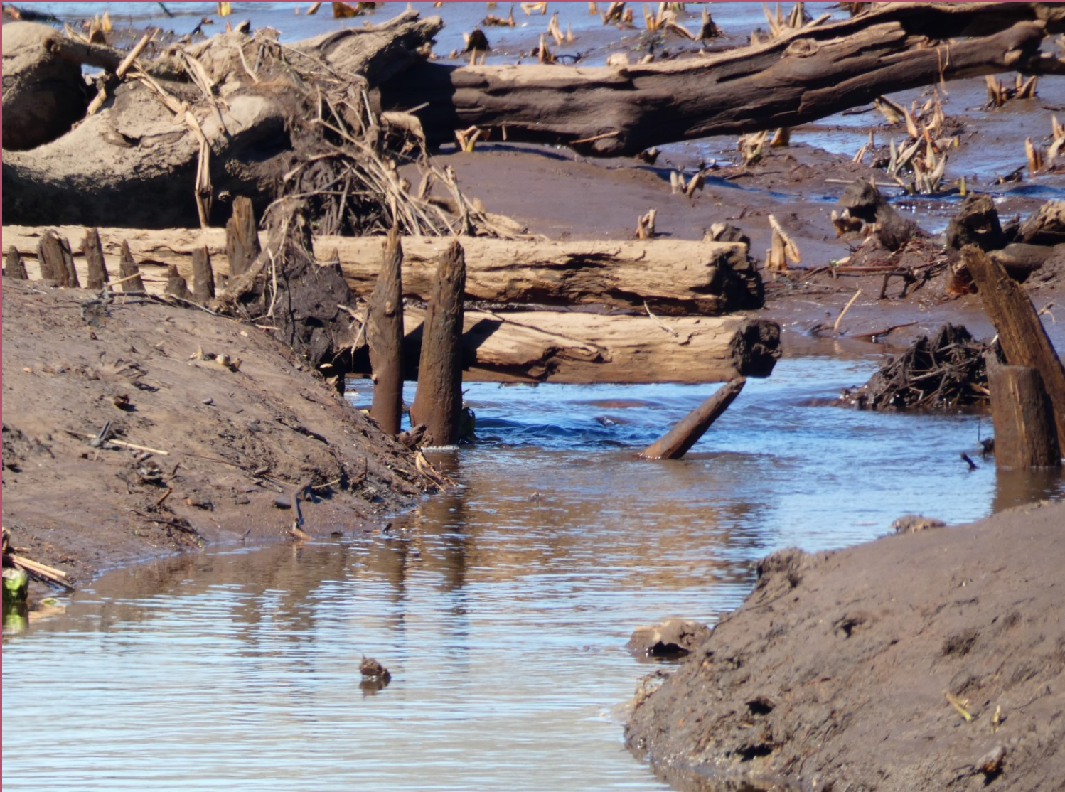
Tide Gates Cast Away Island
