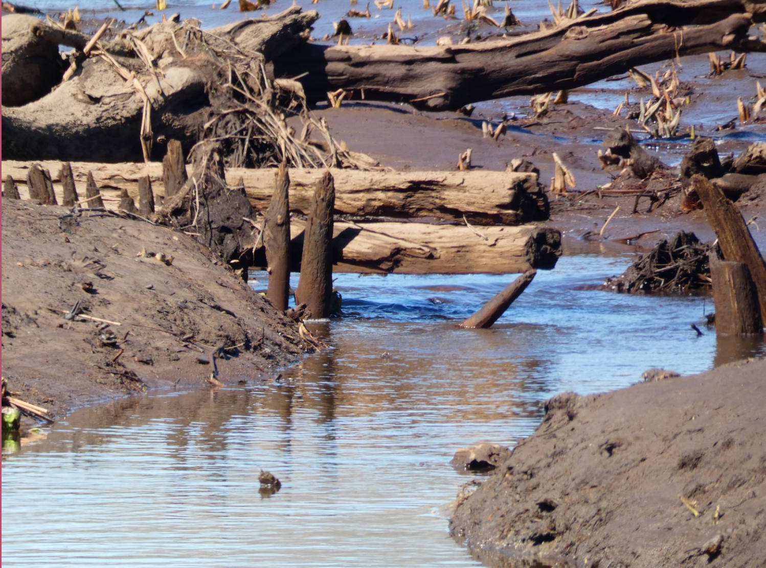
Tide Gates Cast Away Island
