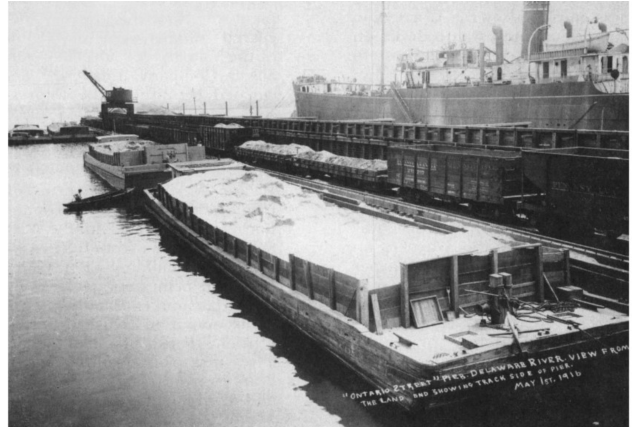
Transportation continues to be a major factor in the sand and gravel business. This 1916 photo is of a Warner pier located at the juncture of the Delaware River and Ontario Street in Philadelphia. Barge loads were transferred to railroad cars, horse drawn wagons and ocean going vessels. The ship in the background transported sand and gravel used for construction in Florida.
